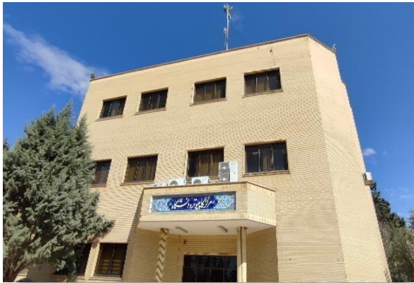
Figure 7. South elevation of computer center building.
