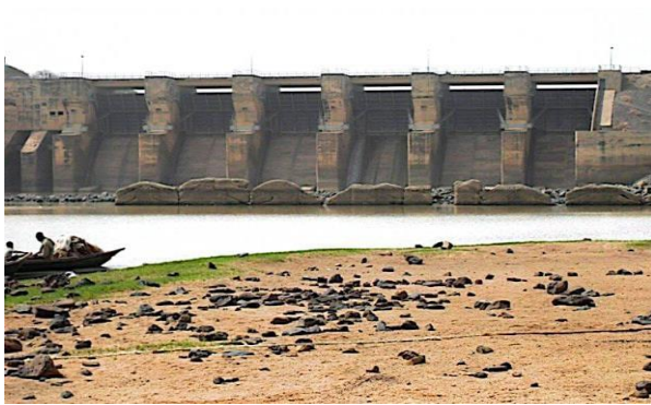
Figure 1. Photograph of Kiri dam spillway and sluices taken by the author during investigation.
